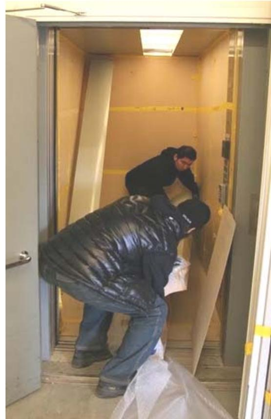
**Figure 4:** Parcel opened and carried into elevator due to parcel design not fitting in-transport route.
