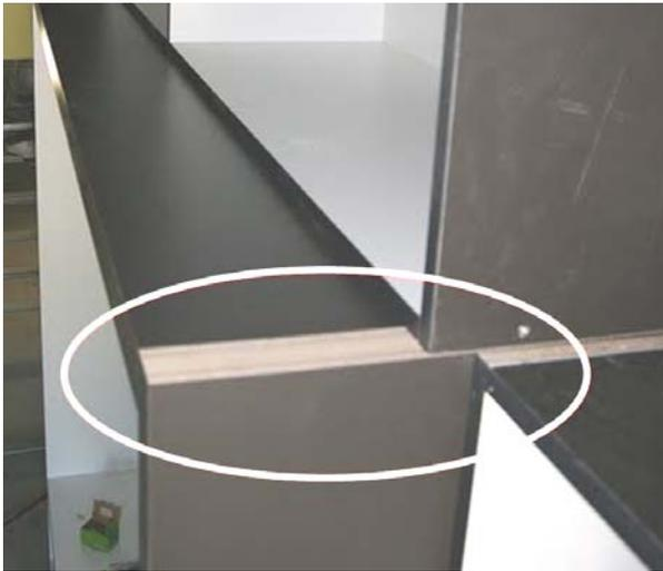
**Figure 3.** Design error, the laminate is missed on the top of the lower shelf.
