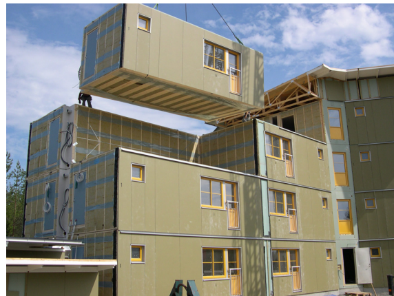
Figure 3. Modular house production.
