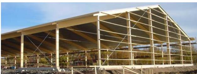
Fig. 2 A long-span timber structure situated in Sweden (only the structural system is shown).
