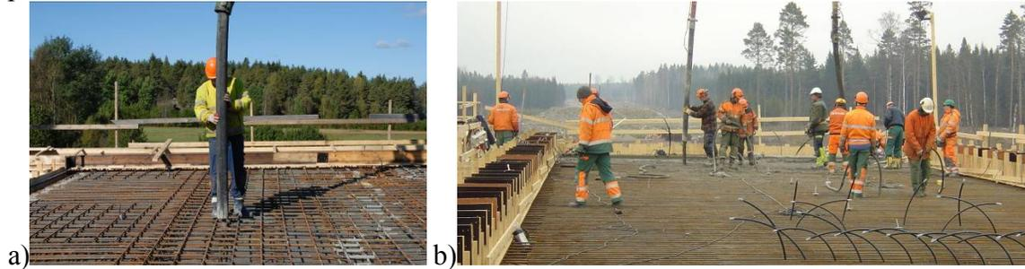
Figure 1: Typical Work Situation When a) Casting SCC. and b) Casting of Normal Concrete
