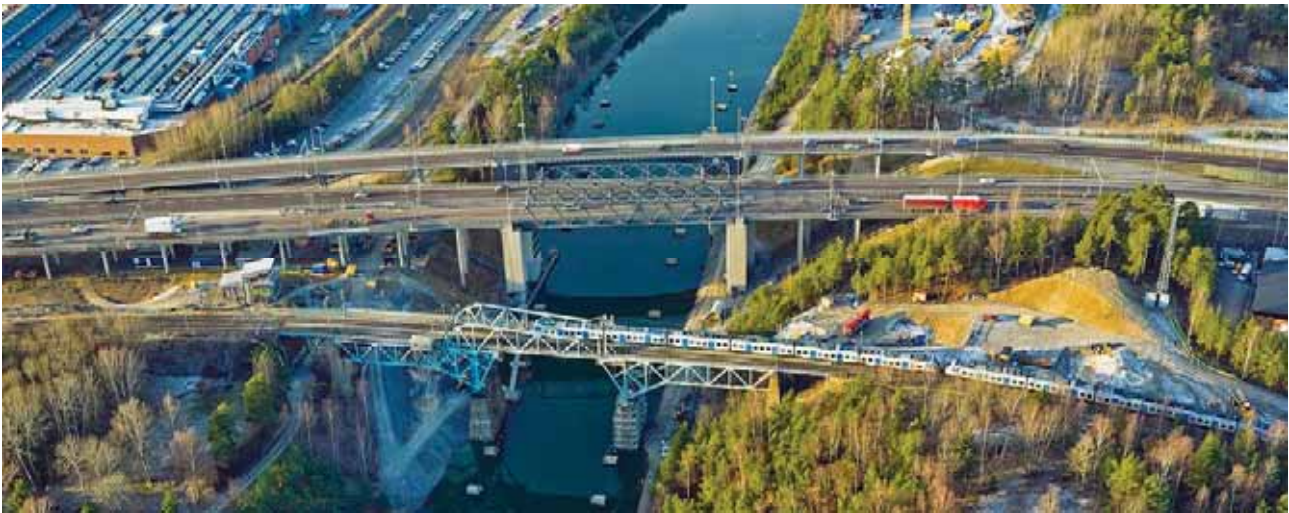
Figure 1. Aerial photo of construction site taken during mobilization.
