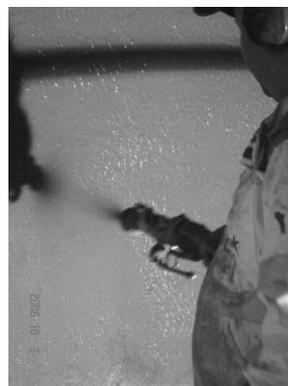
**Spraying mortar onto the pre-mounted CFRP grid**
