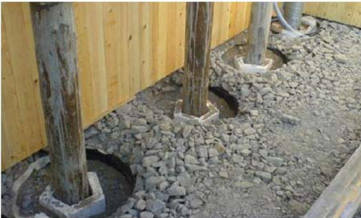
Figure 1. Piles are wrapped with Styrofoam.
