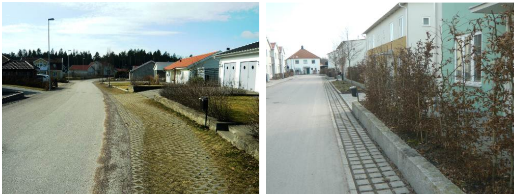
Figure 2. Views of two of the sites: infiltration system with vegetated CGP (left) and ICP filled with gravel (right)
