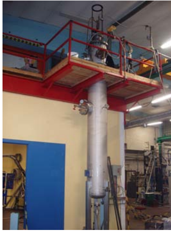
Figure 1.6: Spray test rig at Energy Technology Centre.
