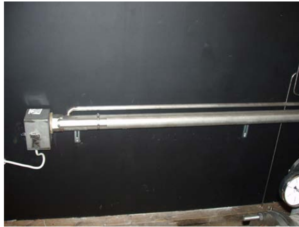
Figure 2.8: 9kW nitrogen gas heater.
