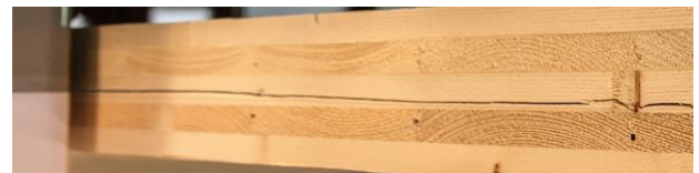
Figure 10: Failure due to longitudinal shear occurred as shear stress parallel to the grain
