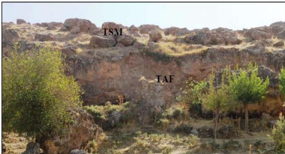
Figure 14: The toe area of the old alluvial fan (TAF) and that of the slid mass (TSM)
