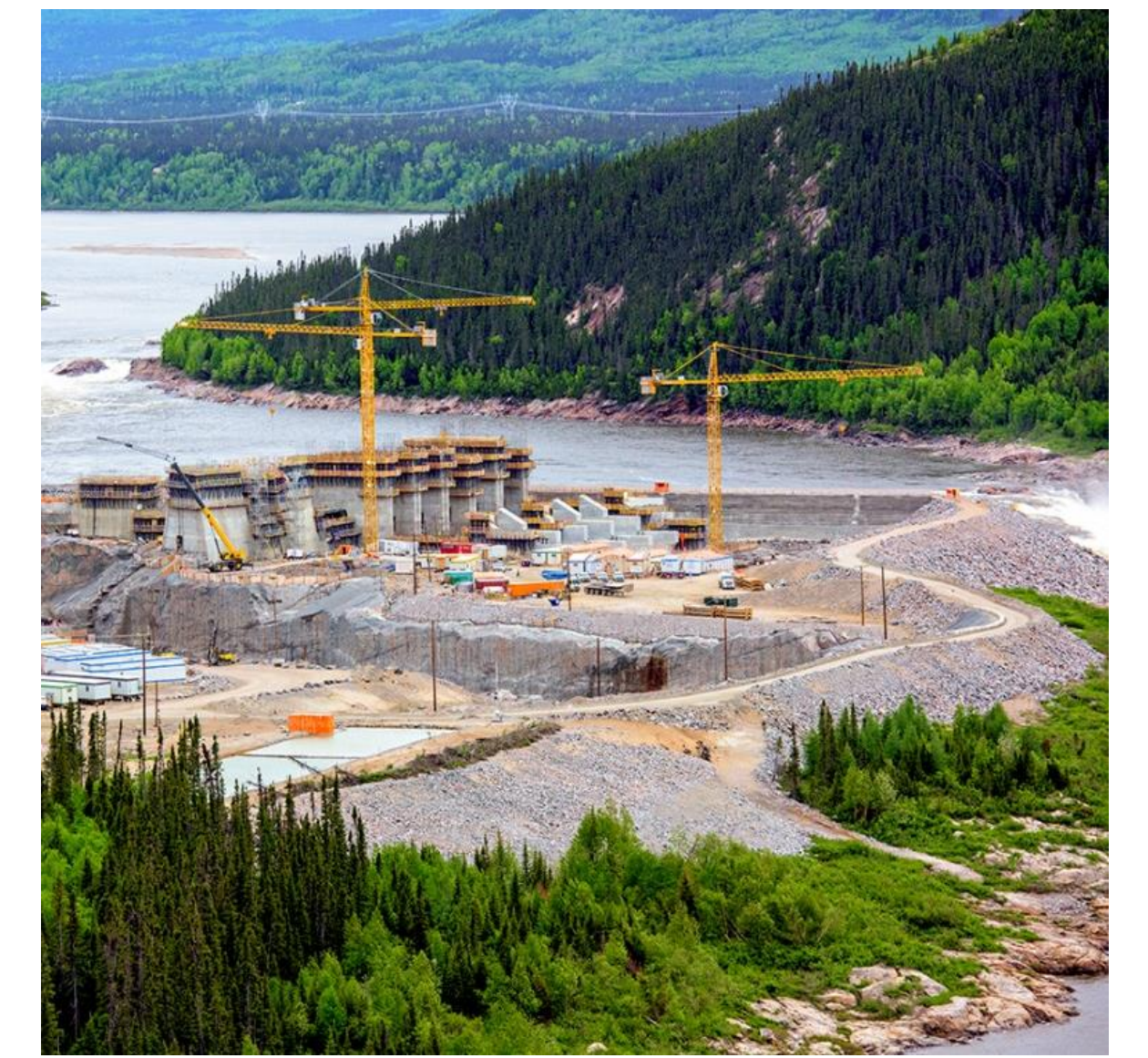
Fig. 2. Construction site at Muskrat Falls http://muskratfalls.nalcorenergy.com/
