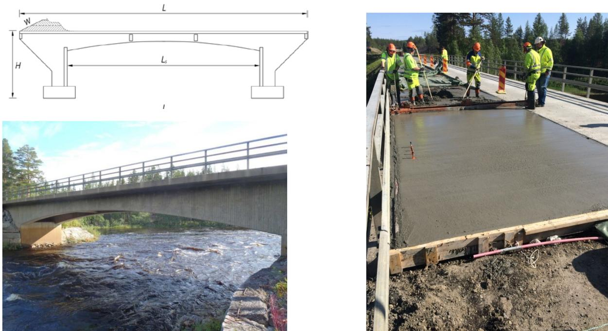
Fig 1. Studied bridge with a span of 25 m and a total length of 37.5 m, bridge deck width: 6.9 m. Concrete overlay casting of one traffic lane.
