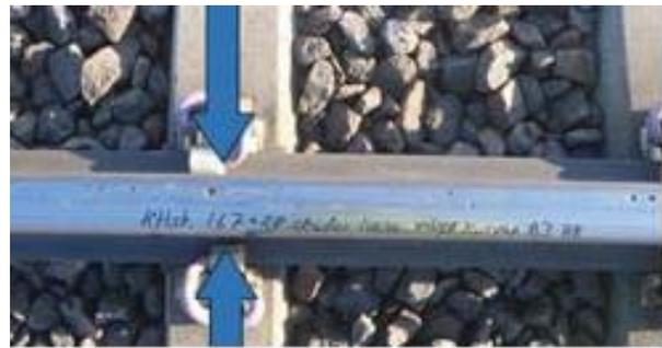
Figure 10. Low rail with spalling on the running surface.
