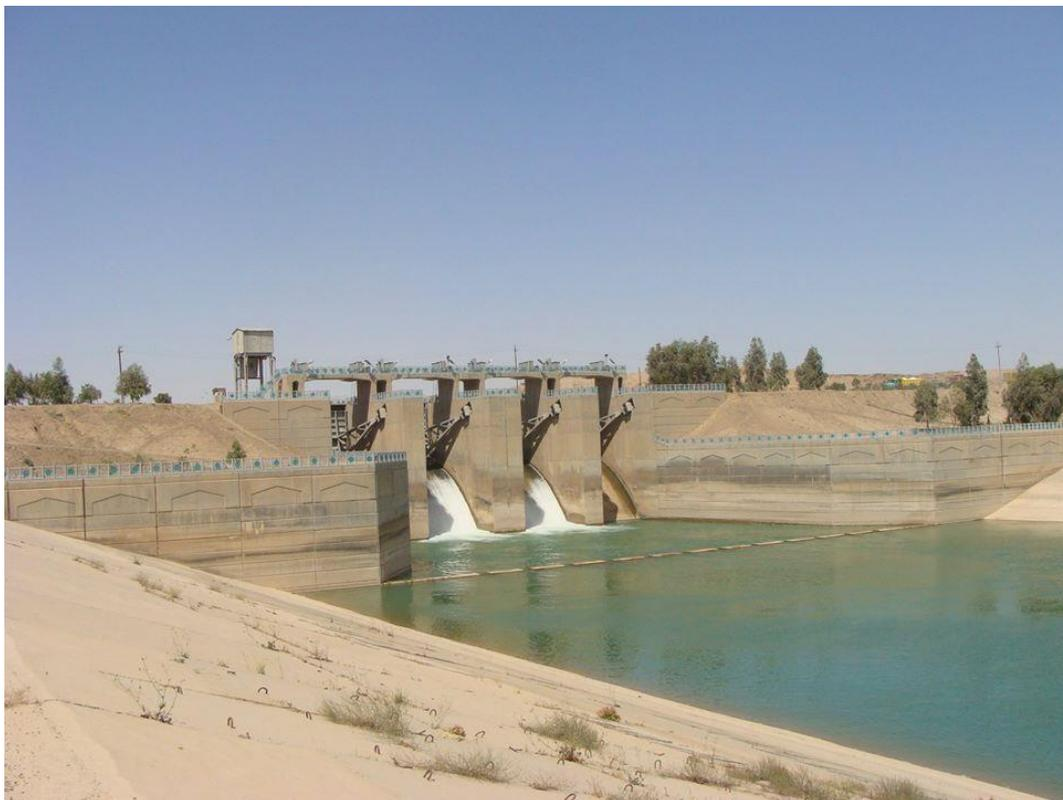
**Figure 6: Downstream view of drop regulator on the Tharthar-Tigris Canal. (Source: [6]).**
