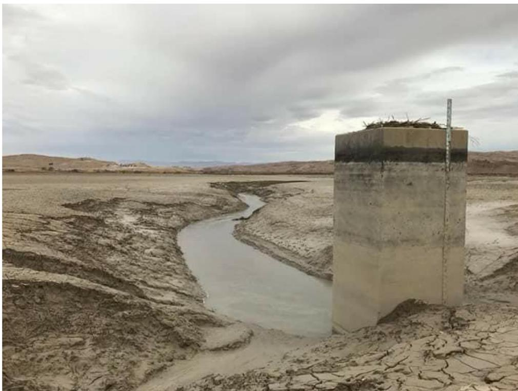
**Figure 2: General view of Mandaly Dam Reservoir filled with sediments. (Source:[7]).**
