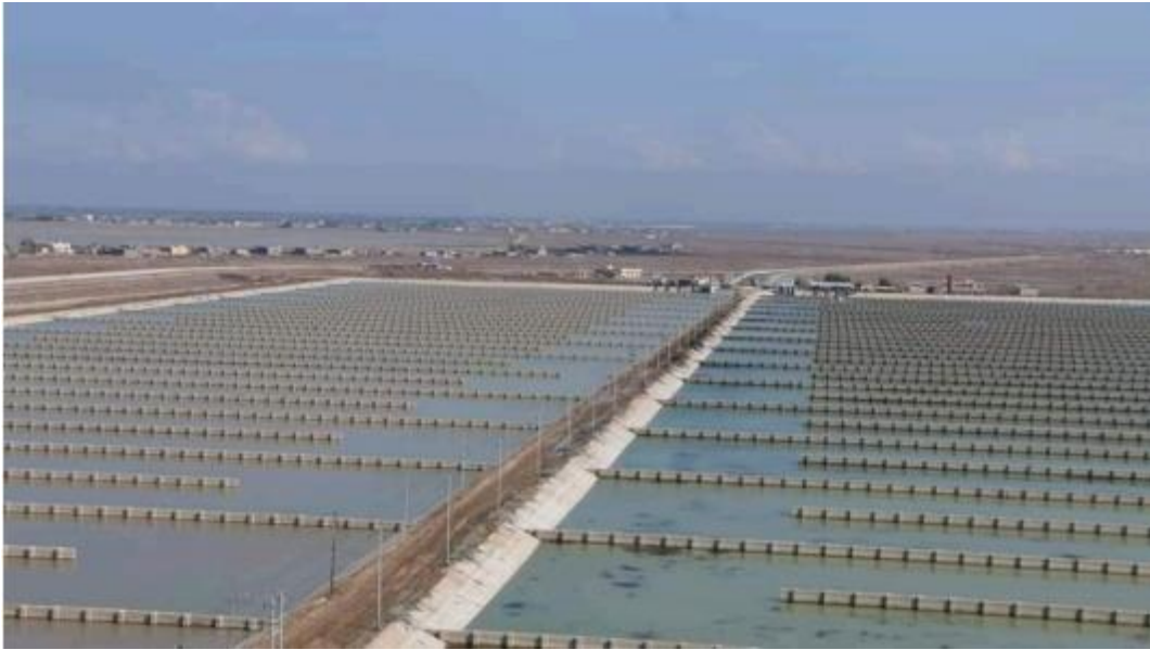
Figure 6: General view of R0 reservoir (Ministry of Water Resources, 2020.)
