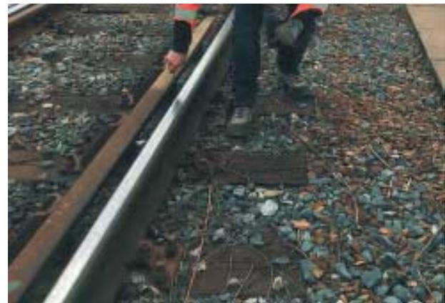
**Figure 6.** Applying friction modifier on the checkrail.
