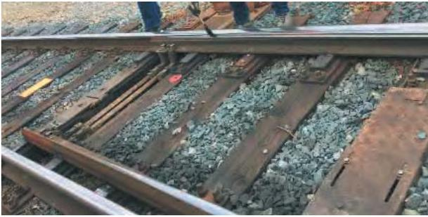
Figure 7. Applying friction modifier on the switch rail.
