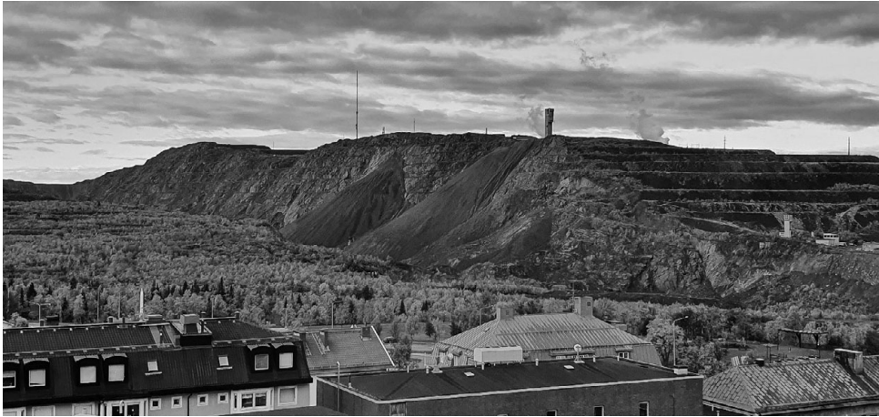
Figure 11.2 Kirunavaara – the mountain where LKAB has been mining for over 120 years, designated as a national interest for cultural heritage preservation by the Swedish National Heritage Board, and an example of the heritage values that the mining operations have generated. Photo by Dag Avango
