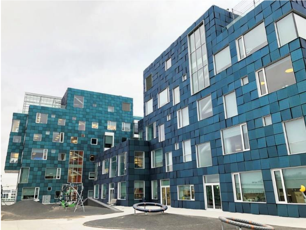
Figure 8: BIPV systems in the facade of Copenhagen International School (Stridh, 2018).
