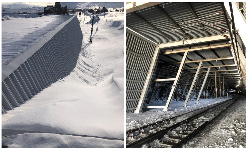
Figure 16. Snow galleries view from outside (left) and inside (right).
