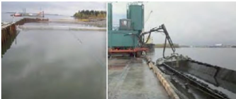
**Figure 2:** On-site pugmill mixing freshly dredged materials with binders (right); the mix was discharged underwater into a reclaimed area (left) (Photo: Courtesy of Port of Gävle)
