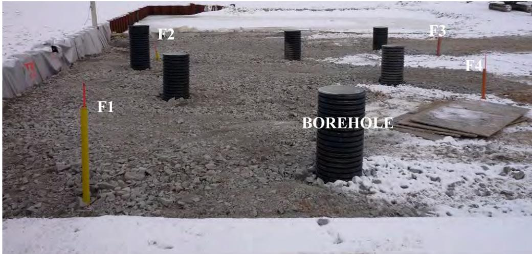
**Figure 3:** Monitoring instruments and preloading layer of selected gravel on finished SCDM fill
