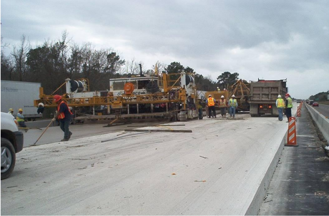
Figure 6. Pouring of self-healing concrete on highway IH-10, east of Houston, USA.
