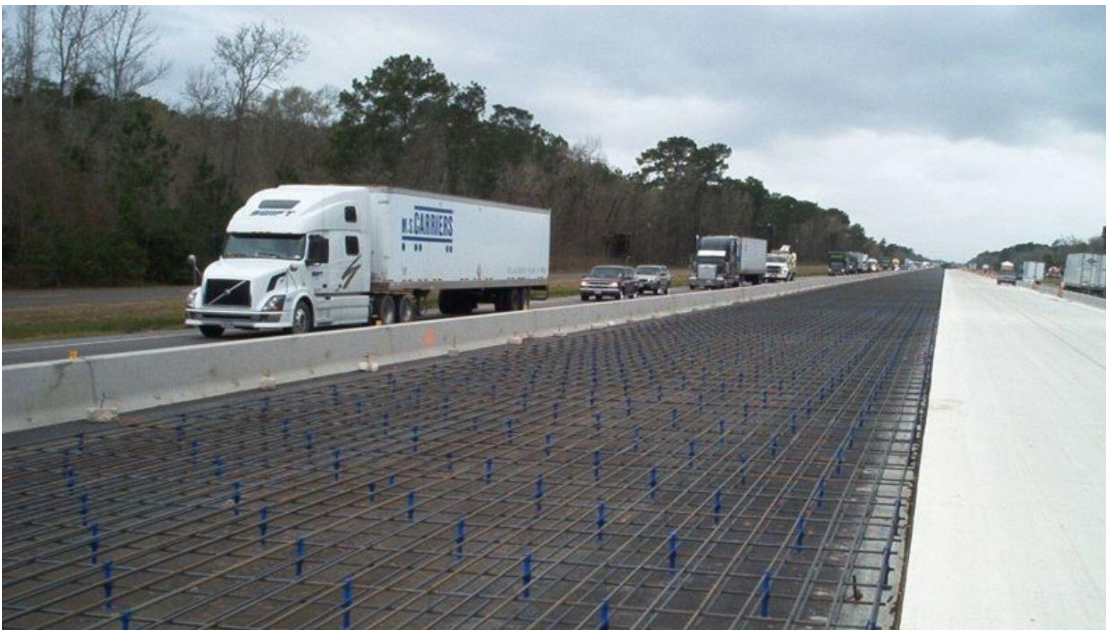
Figure 7. Reinforcement ahead of concrete placers on IH-10, east of Houston, USA.
