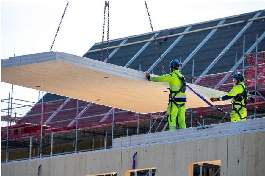
Figure 1. Assembly of a CLT flooring panel. Photo: ByggPartner i Dalarna AB.
