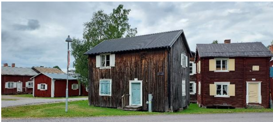
Figure 11. Street view of a church cottage in Öjeby Church Town showing a newly installed sheet-metal roof, illustrating recent material replacement within the historic built environment. (Photo: Author).
