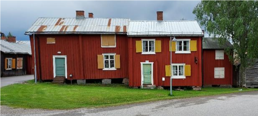
Figure 10. Street view of Öjeby Church Town showing traditional church cottages with later sheet-metal roof replacements, reflecting incremental material changes introduced during 20th-century renovation practices in the heritage environment. (Photo: Author, based on Öjeby Church Town building documentation, Piteå Municipality)
